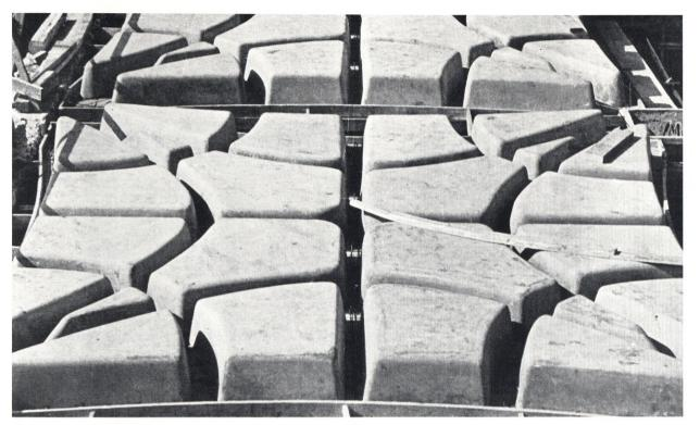
Detail of prefabricated ferrocement formworks
