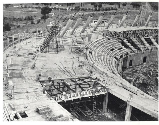
Construction of the Palazzo dello Sport, Rome, 1959, detail of floor with isostatic ribbing
